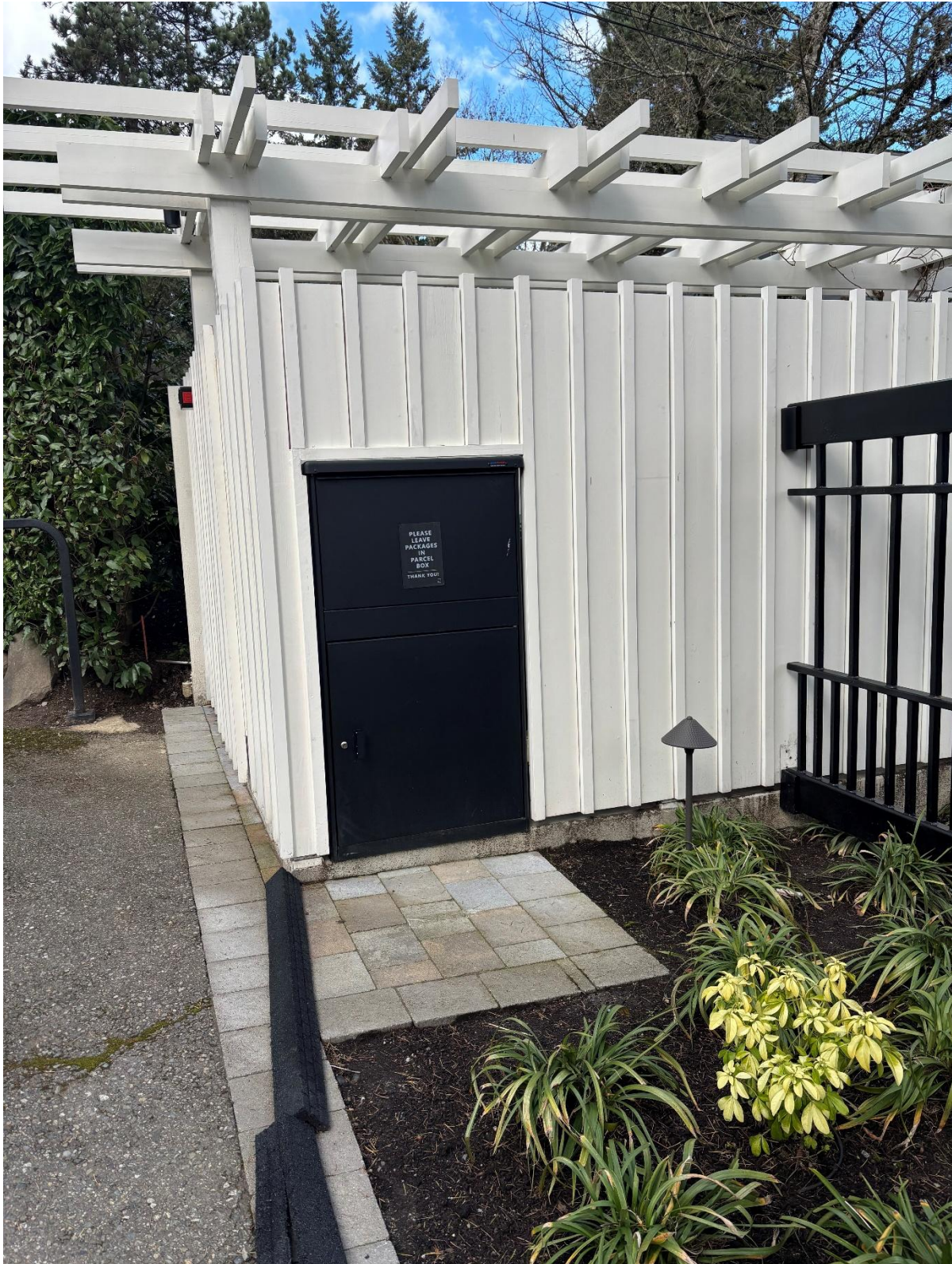
View of parcel locker from southwest
